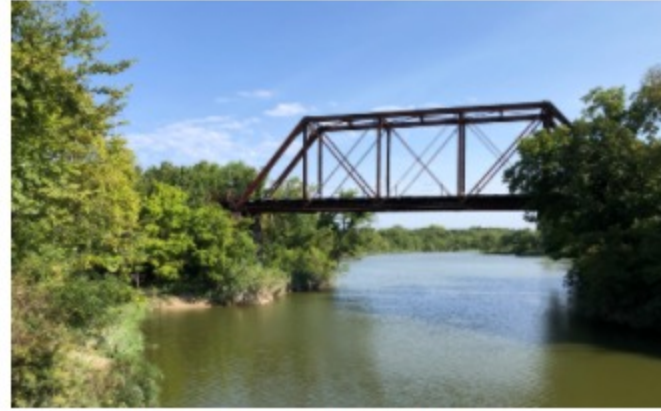
The KCS Railroad Trestle over White Rock Creek
